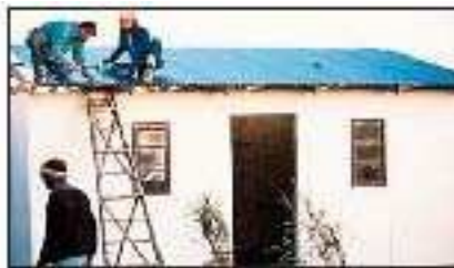
Detailing Window Setting Roof Panels
