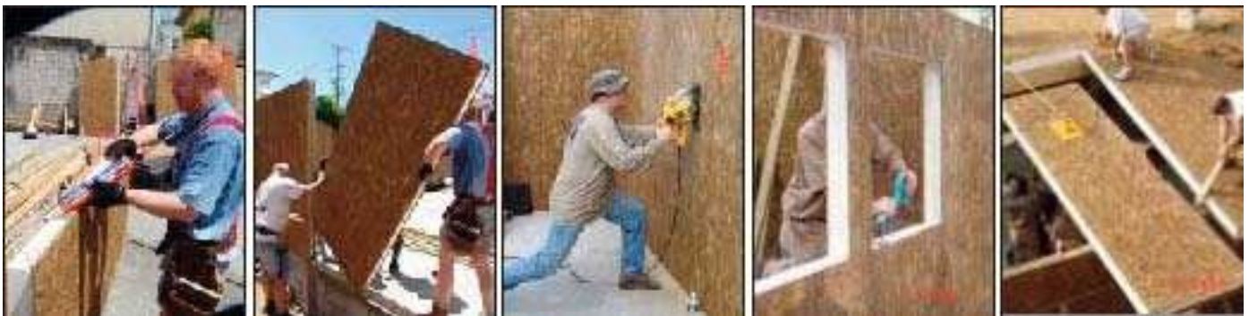
Prepping SIP Panel Standing Wall Panel Cutting in Window
